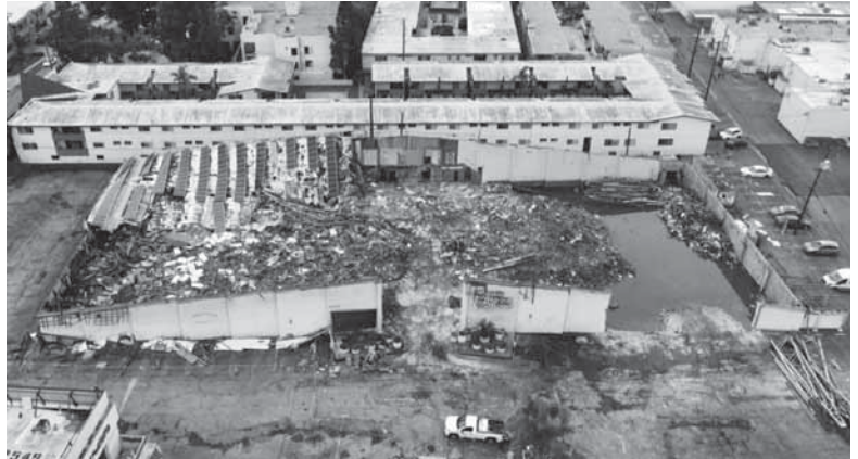
Gable House Bowl Demolition
